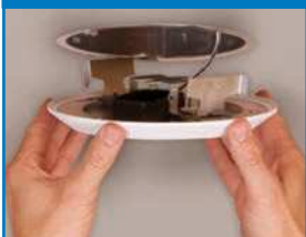
6-inch friction clip position
