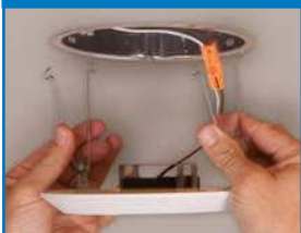
6-inch torsion spring position
